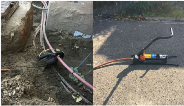
Fig. 47: Cutting plyer used to perform an earth fault
