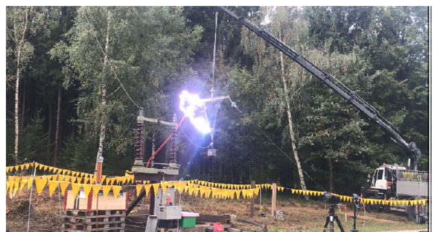
Fig. 37: Artificially triggered earth fault in a 110-kV-network
