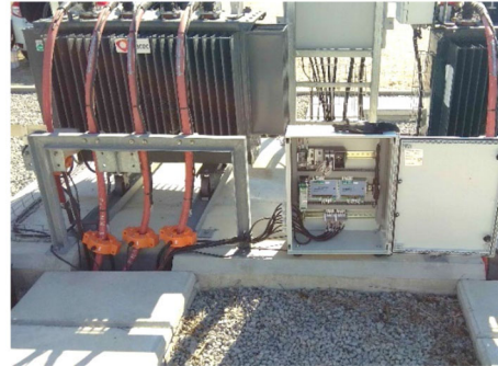
Fig. 2 of paper 526: Easy-to-install split-core current transformers on a grounding transformer.
