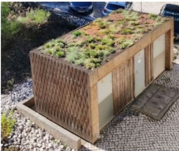
Fig. of paper 617: Smart Substation Eco-housing with usage of cork.
