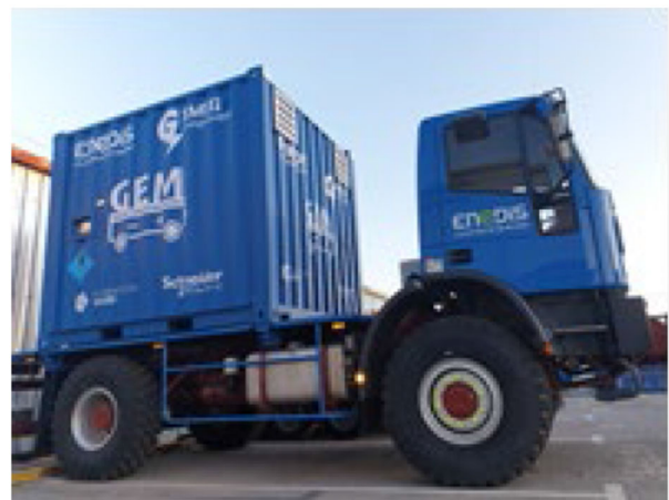
Fig.6 of paper 890: “GEM” generator on a truck
