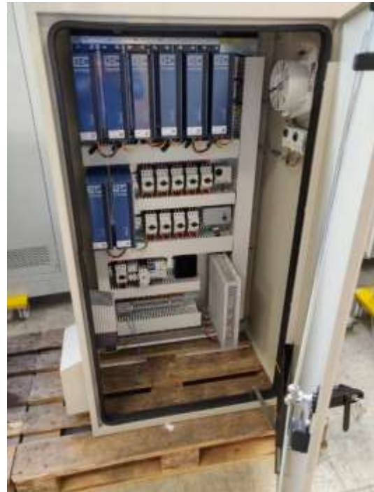
Figure 3.3-28: N470 Outdoor substation for public lighting.
