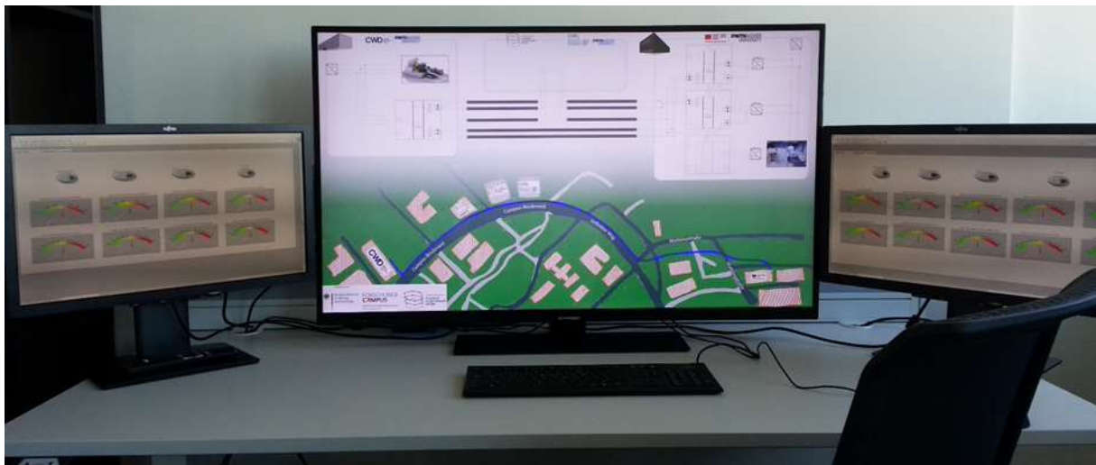
Figure 3.4-26: Control station at FEN Research Campus.
