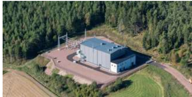
Figure 3.4-18: Åland converter station.
