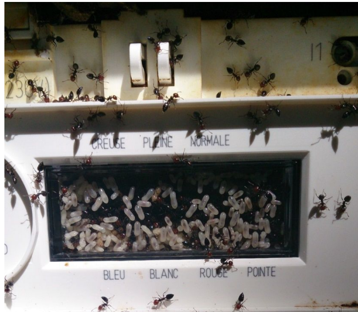
Figure 3: Example of a meter infested by ants
