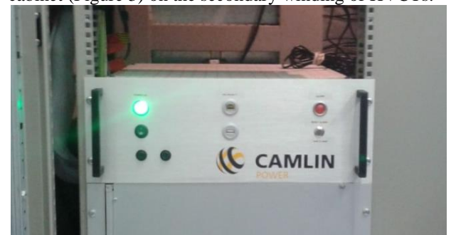
Figure 2: TFC monitor installed in TERNA control room
