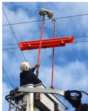
Figure 7 Mounting of line sensors
