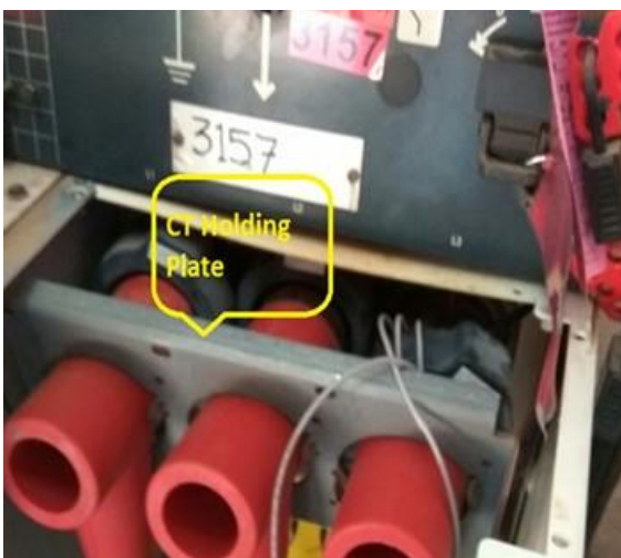
Fig:-2 CT holding plate installed on RMU bushing
