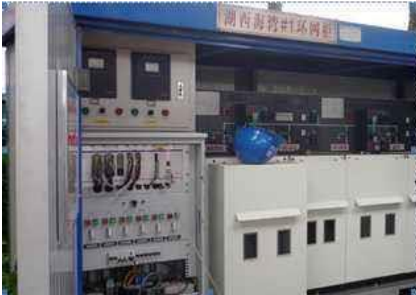
Figure 5 Installation of the STU at the 10kV ring main unit
