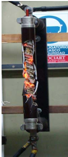
Figure 6, Laboratory test of a low current operation failure of an aged HBC fuse.
