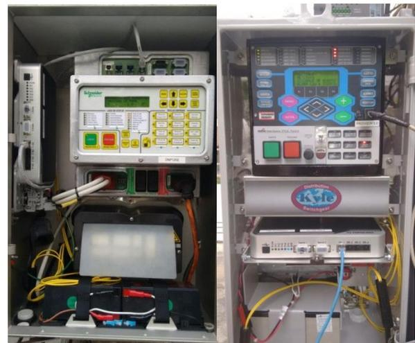
**Figure 12.** Reclosers controllers Schneider ADVC2 panel (left) and Cooper Form 6 (right) with Fibermesh.
