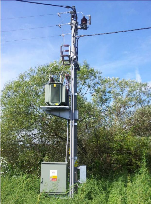
Fig. 2 Substation MV/LV Jarohnevice with the transformer FITformer REG
