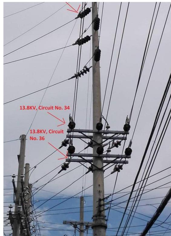
Figure 1 – A picture of the network arrangement at Dagupan Electric Corporation, Philippines.
