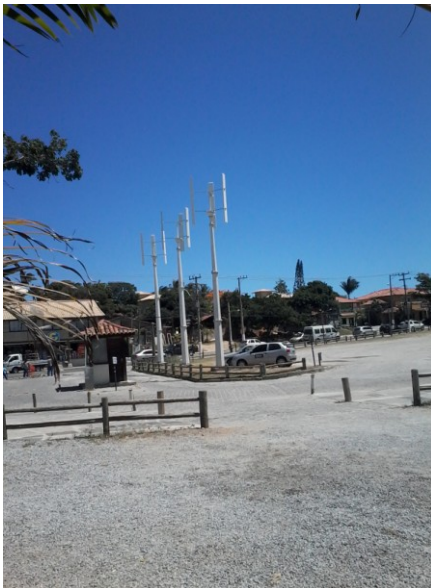
Figure 5. Vertical axis wind generators
