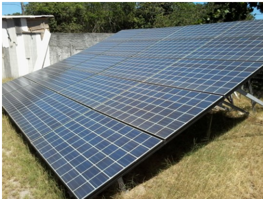
Figure 1. Polycrystalline film panels installed in APAE (a Brazilian public educational institution devoted to children with special needs)
