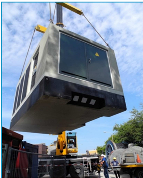
Figure 7. Prefab MV/MV substation being placed
