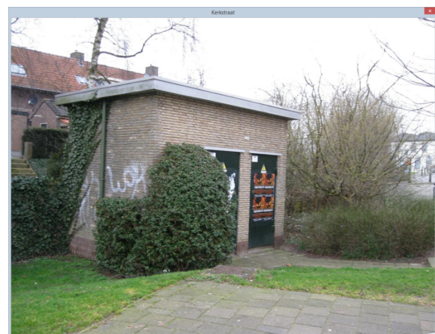
Figure 8. Picture of substation
