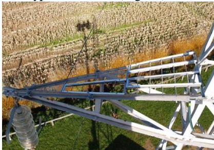
Fig. 16 - Oblique Structure for metal poles
