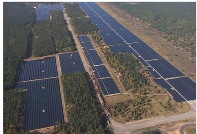
Fig.6 Solar Energy production in Groß Dölln ca. 140 MW
