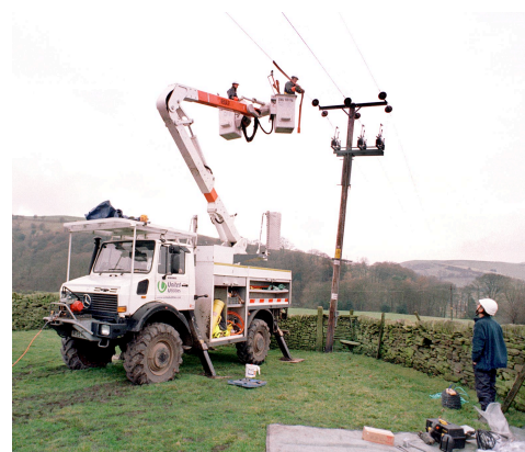
Figure 4 Live Line Working Techniques
